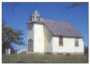
St. Oswald was built in an unusual manner: with a wood framework and grout walls, grout being a combination of lime and sand. The interior finish was lath and plaster.
